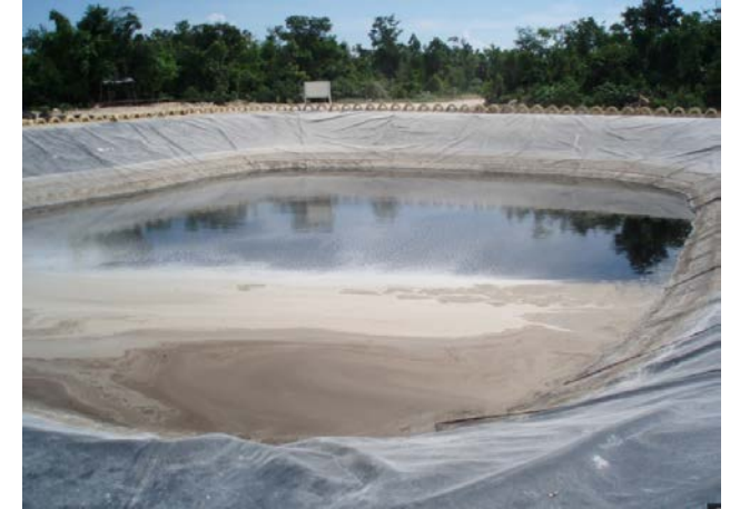
Lined Evaporation pond
